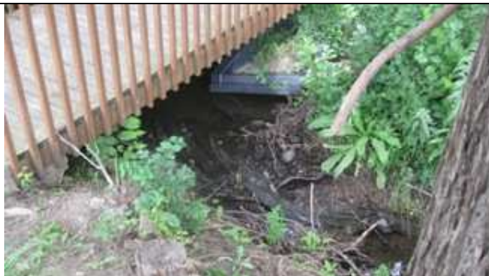
Washout Under Walkway Bridge at Ellsworth Rd.
